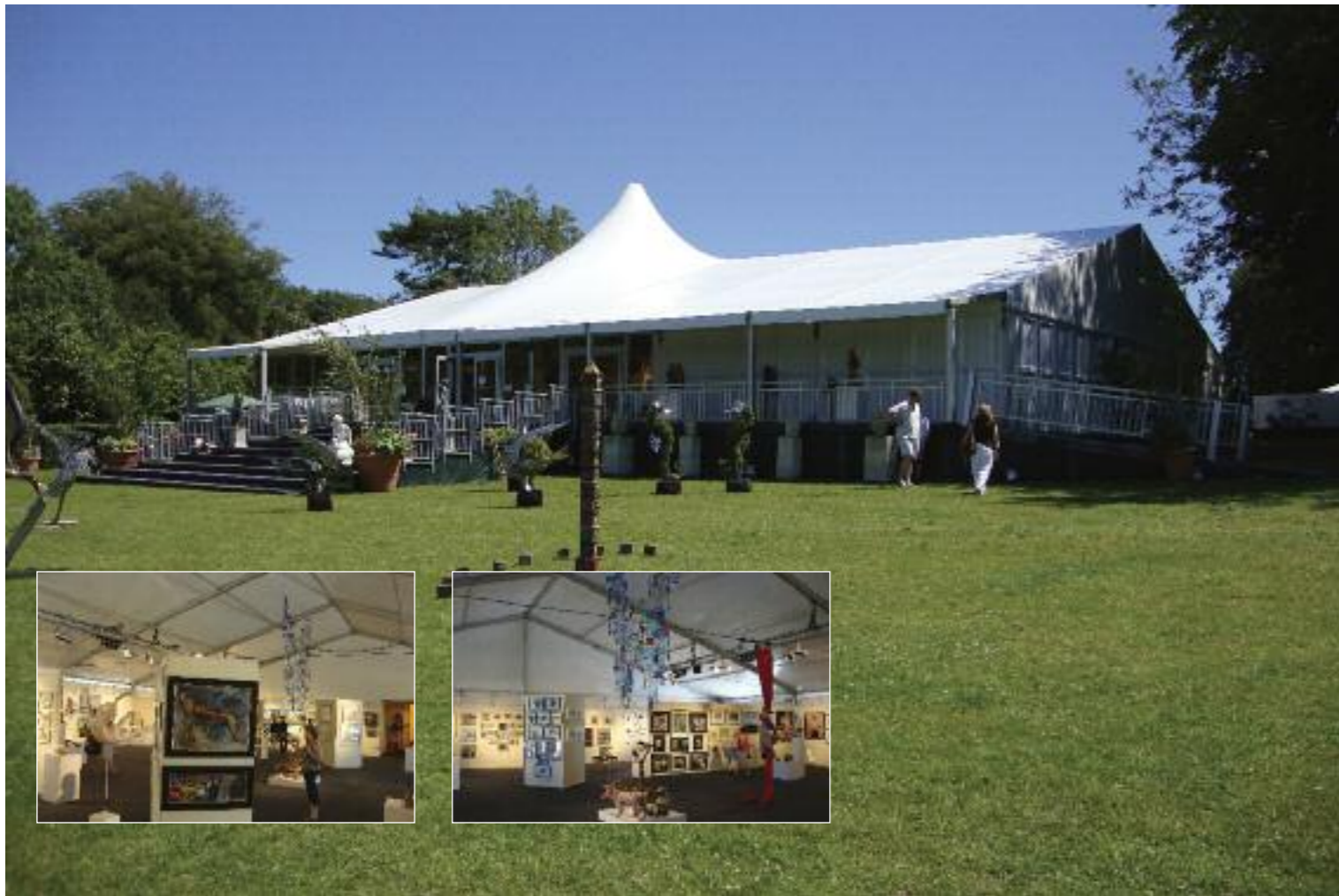
21M X 25M WITH DOME PEAK ROOF & 3M ANNEX CUSTOM BUILT STUD WALLING/INTERNAL PARTITIONS AND STAIRS – HAMPSHIRE
